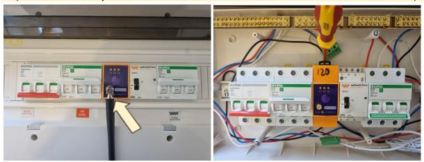
**STEP 2** Remove the green plugs on the top and bottom of the Auditor device. You should **NOT** need to undo any screws during this operation.
